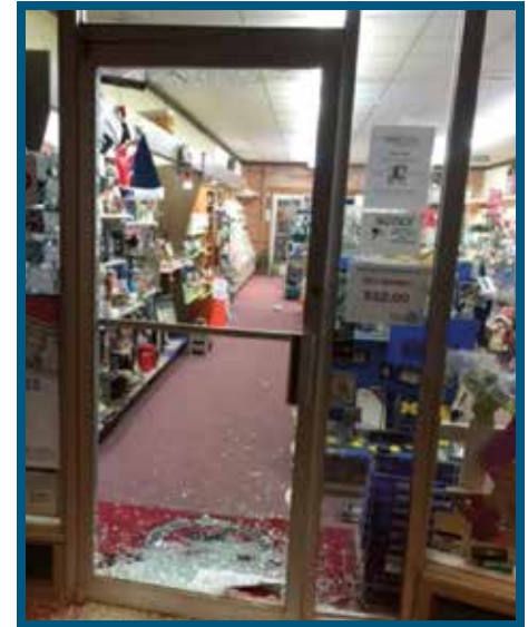
The preferred route of entry for almost half of pharmacy burglaries is through the front door.
